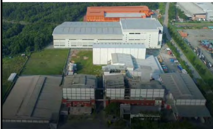
Figure 4: JP Foods' first cocoa-processing plant in PTP, Johor, Malaysia
